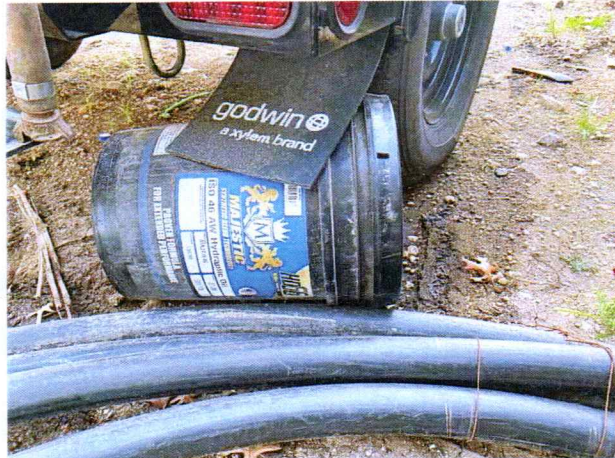
Spilled Hydraulic Fluid in Material Storage Located in NDZ
