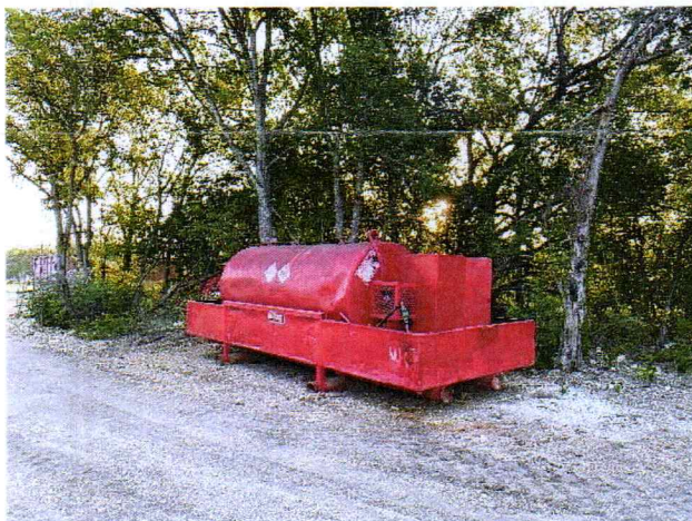
2,000 Gallon Liquid Fuel Tank Located in NDZ
